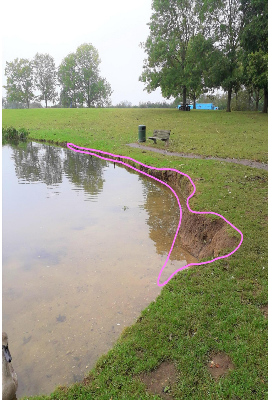
Photo 2 - Stretch of river bank at Caley Green (looking South-West) showing areas of eroded bank (and extent of existing but decaying wooden revetment)
