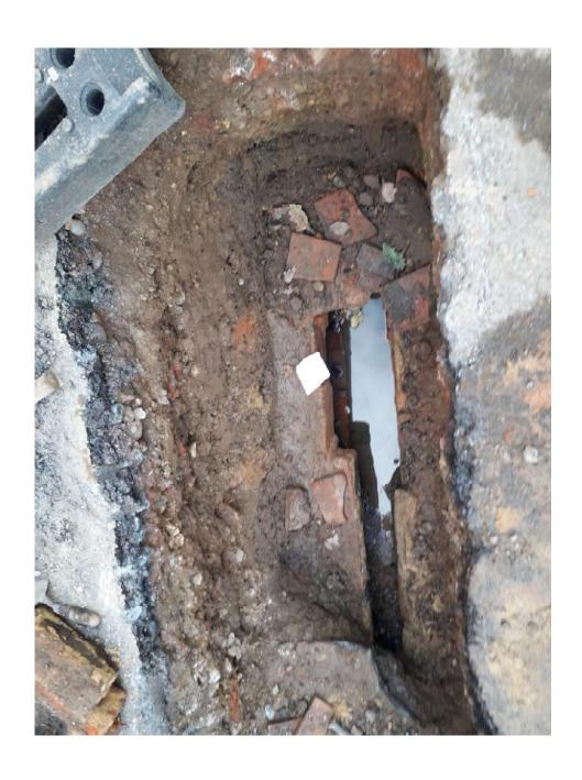
THIS ONE IN BIRCH STREET WAS REPAIRED TEMPORARILY IN AUTUMN 2021 BY INSERTING A PLASTIC PIPE
