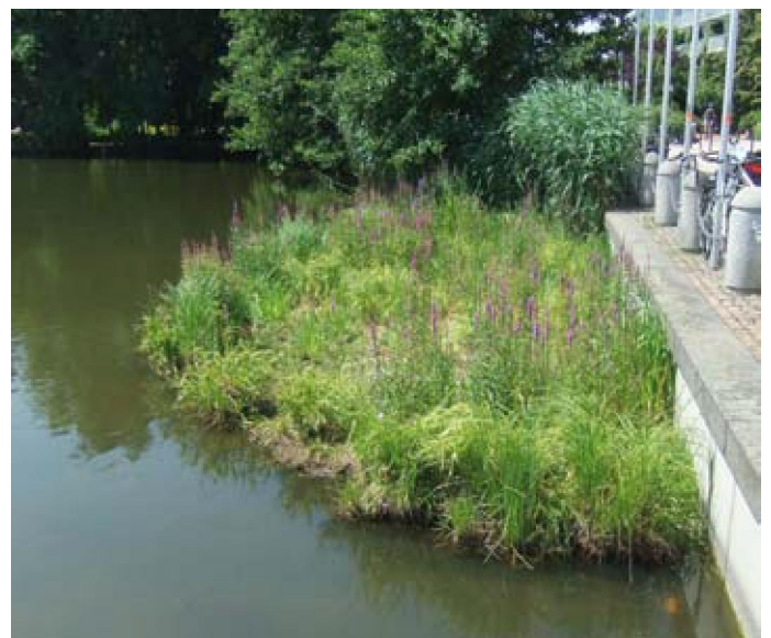
Soft bank protection - establishing well
