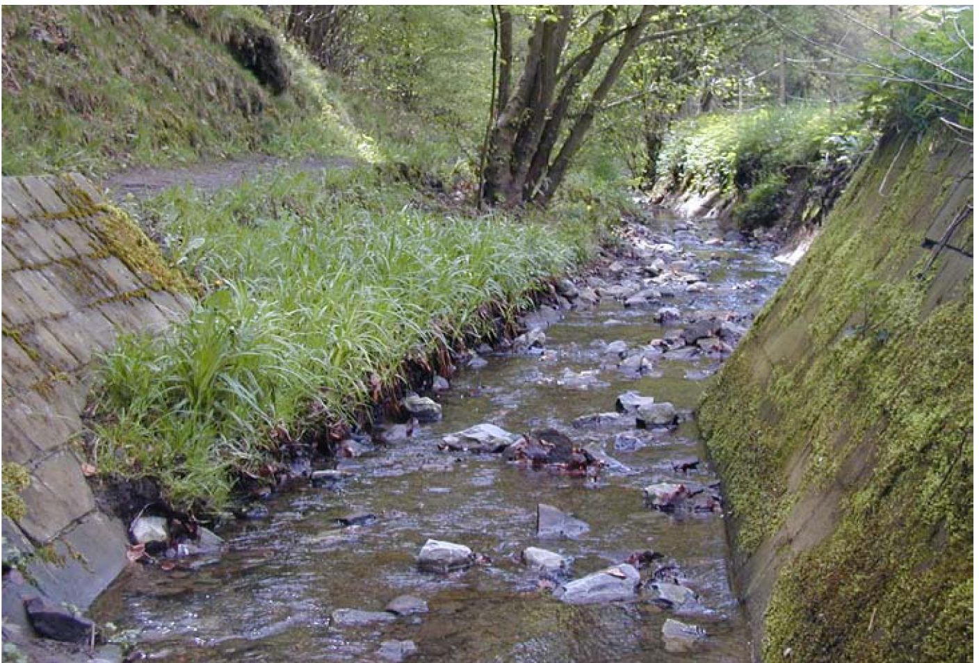
Aqualogs providing robust green revetment replacing hard engineering
