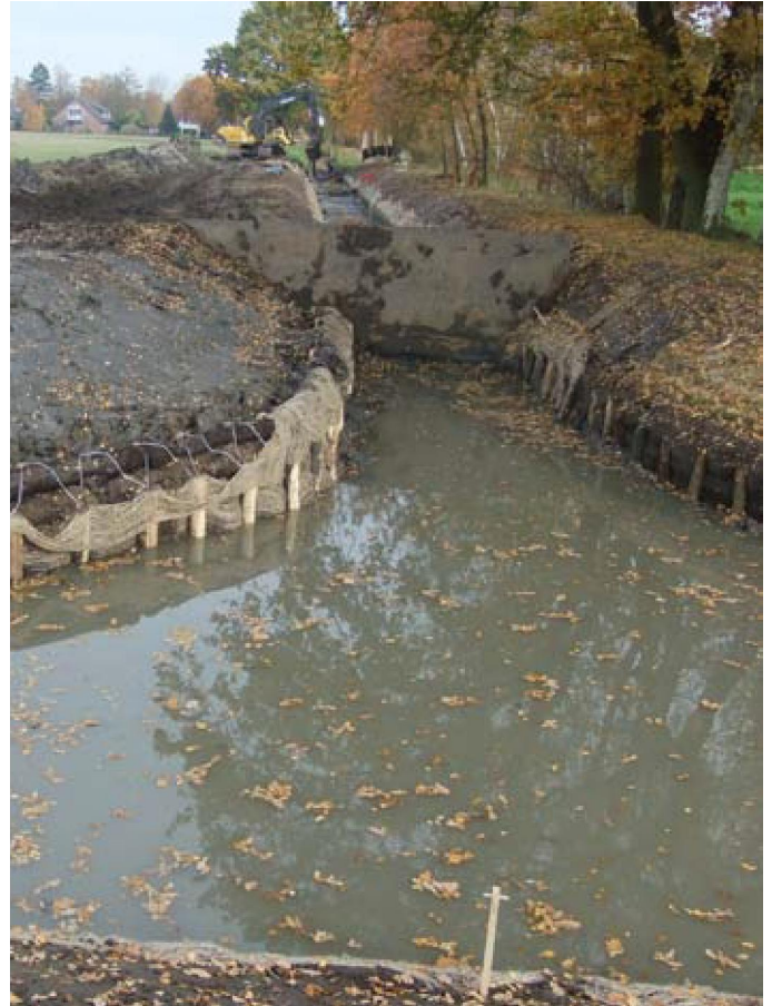
Aqualogs creating a stable bank that will rapidly vegetate naturally
